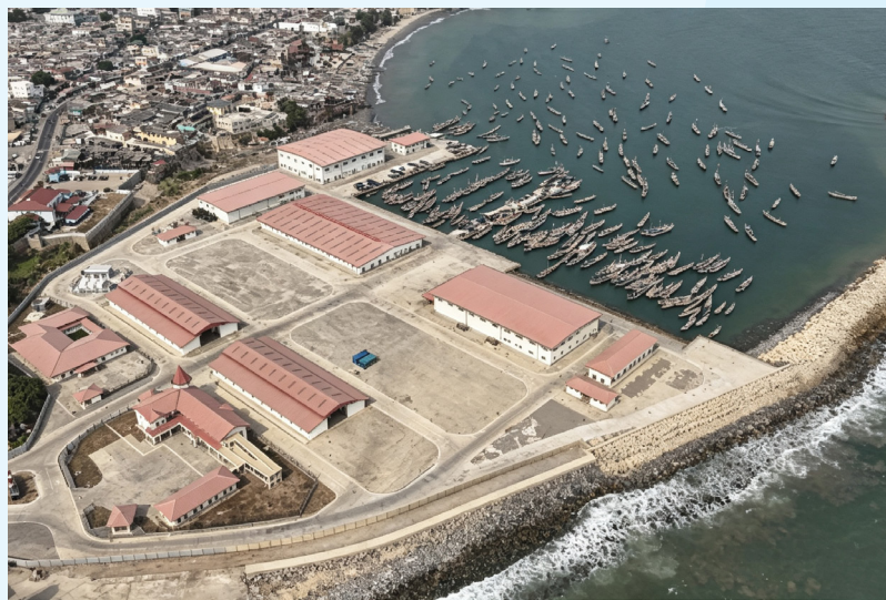
Aerial photo of the Jamestown Fishing Port after construction
