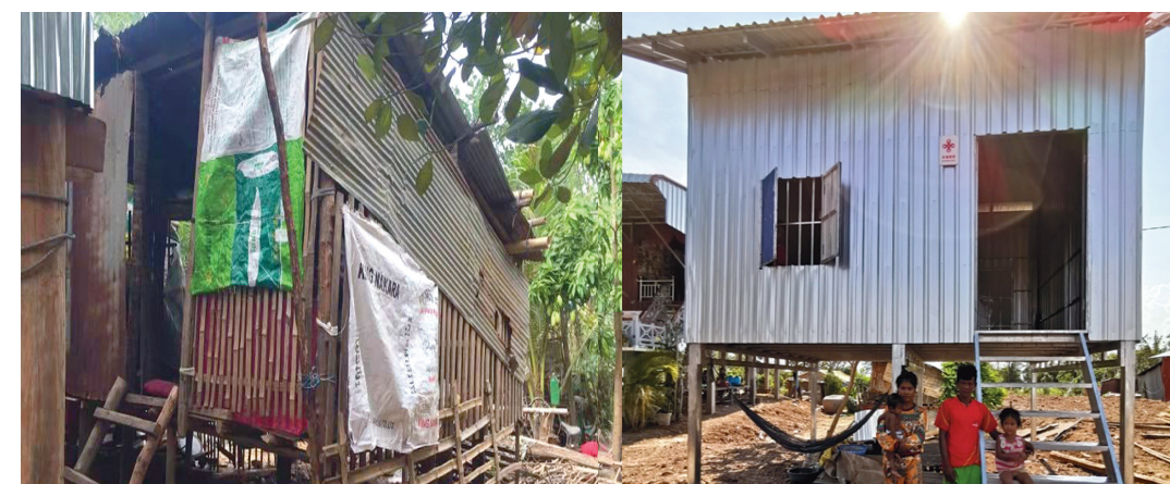
Old and new houses of poor households in the Cambodia project village.
