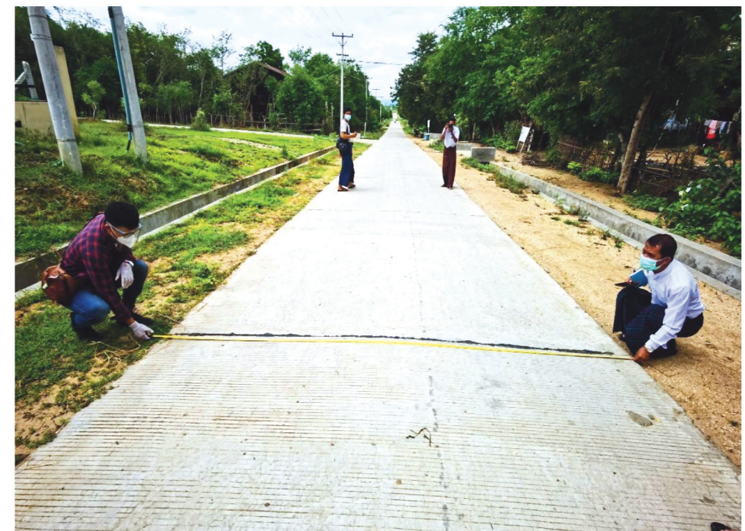
Rural roads repaired by the Myanmar Project.
