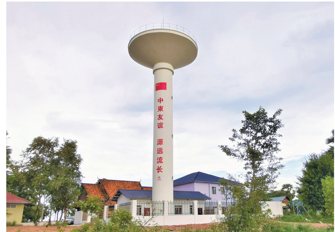
The main tower of the water supply project constructed by the Cambodian Project.
