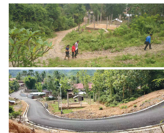
Before and after road hardening in Ban Xienglorm Village, Laos.
