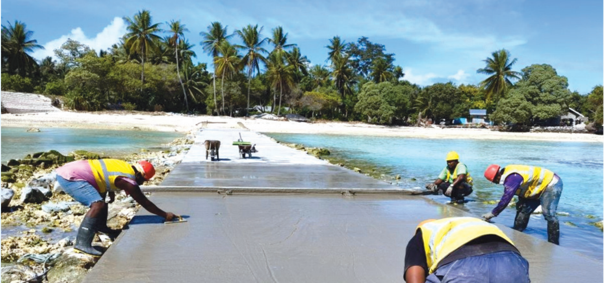
Road surface under construction at Tarawa bridge, Kiribati
