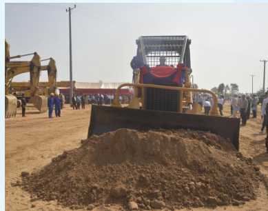
The China-aided Dang Kambet Reservoir Development Project in Cambodia officially begins construction
