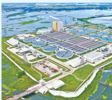
The Dasherbandi Sewage Treatment Plant (DSTP) project built with Chinese assistance
