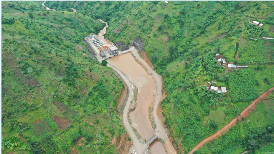
China-aided Ruzibazi Hydropower Station in Burundi
